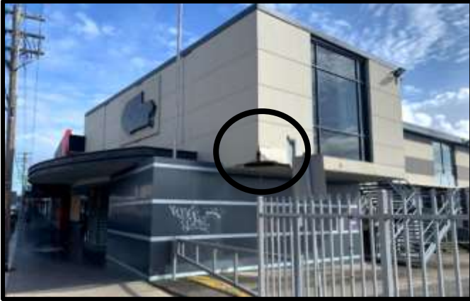
Image 1: Depicts the front view of the site. The site is a two-level structural dwelling used for commercial purposes. There is a vent coming out of the structure. In addition, there is an area which is eroding (seen from circle).
